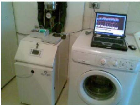
**Photo 2:** The geothermal heat pump (left) and the monitoring system
